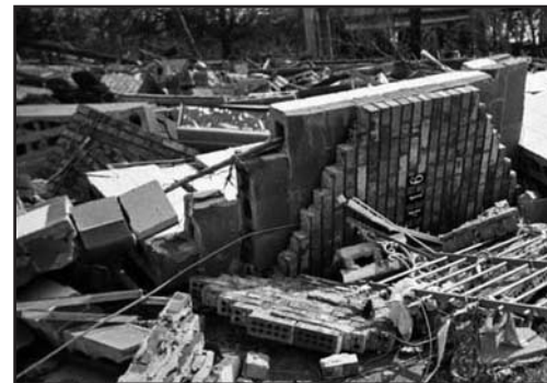
Hurricane Katrina destroyed the Mississippi Coast Chamber of Commerce
