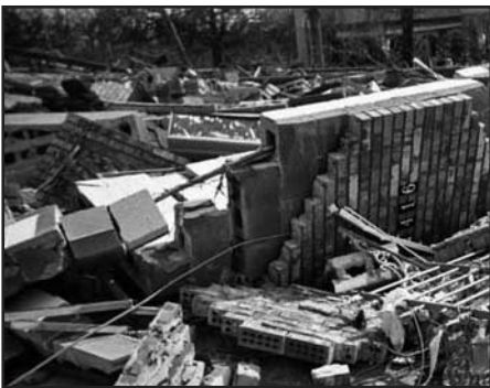
Hurricane Katrina destroyed the Mississippi Coast Chamber of Commerce
