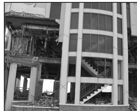
Biloxi Bay Chamber of Commerce decimated by Hurricane Katrina
