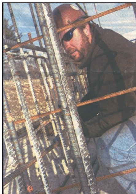
Joseph Holland of Whitman, co-owner of GRC Steel Construction, works with rebar along the back wall of the Ikea store in Stoughton
