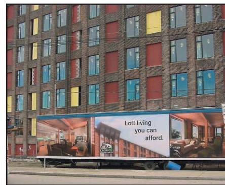
Etonic Lofts, 148 Centre Street, Brockton, MA 02301 Proposed Units: 64 Condominiums Status: Under Construction
