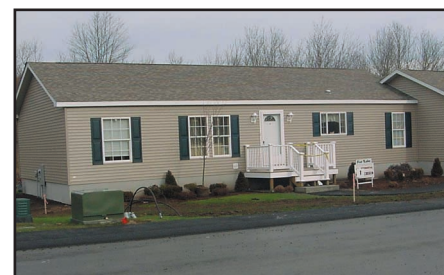
Skyview Village, 2013 Main Street, Brockton, MA 02301 Proposed Units: 60 Senior Residential Homes Gated Community Status: Under Construction
