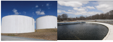
Desalination Plant; Sewer Plant
